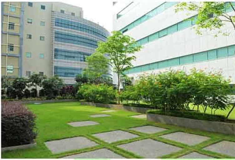
Fig 1.2 Starhub Green Roof Garden at Ubi Avenue 1
